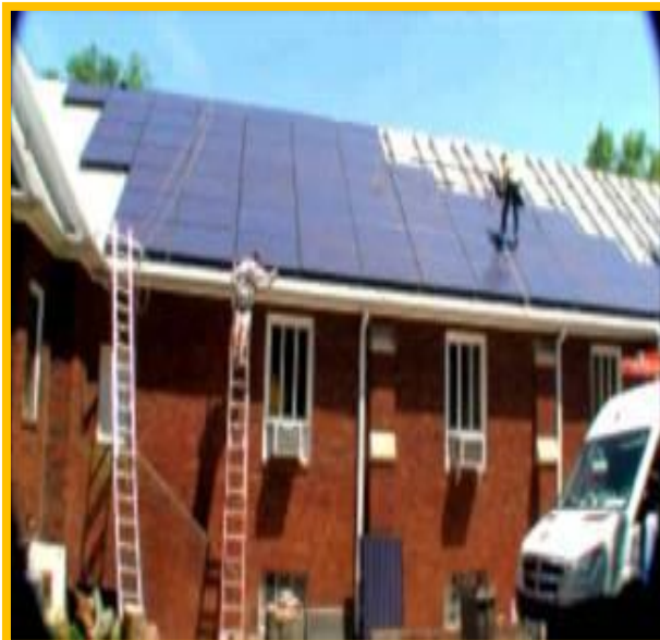
Figure 18: Installation of solar panels on the University Park Church of the Brethren Source: Examiner.com
