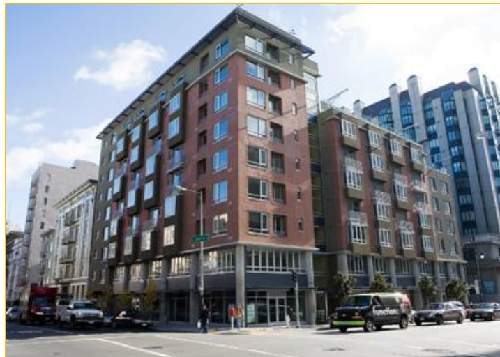
Energy efficient senior and supportive housing in San Francisco, CA
