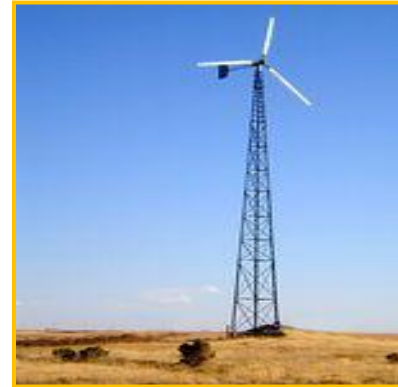
Figure 16: A small wind electric system called the Jacobs 20-kilowatt turbine can provide electricity for a variety of electrical needs from home heating and lighting to water pumping for livestock. Source: NREL.gov
