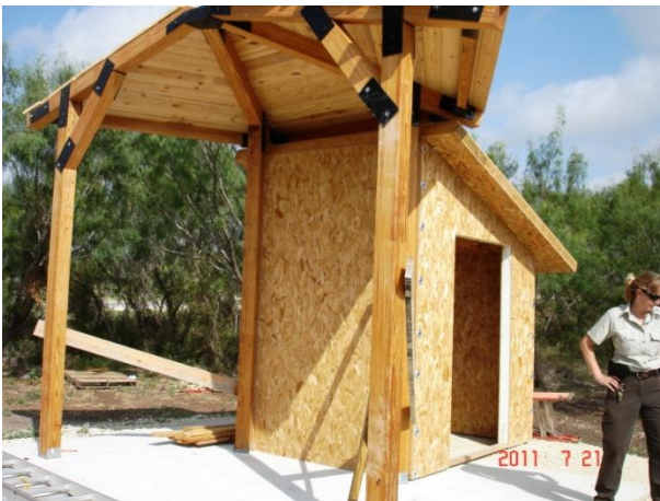
Karin Eldridge and the Outdoor Classroom under construction.
