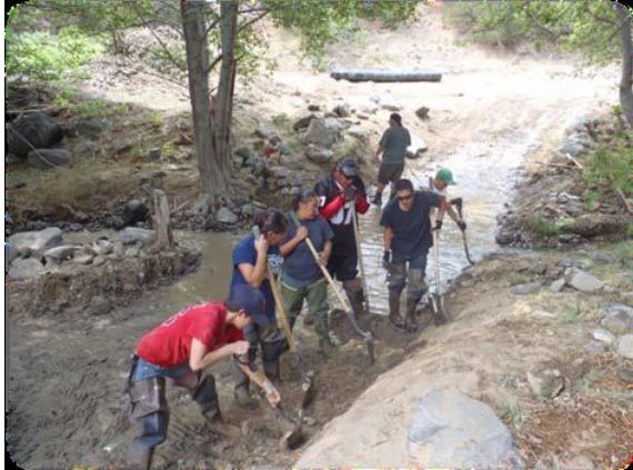
Fish passage crossing construction on the Rio Paguete.
