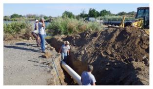
new drain line allowed us to maintain flow into Oster #1 then divert water through the new line instead of into lakes #2-5. This resulted in the ability to drain lakes #2-5 while maintaining full flow to Oster#1 while maintaining suitable temperatures for continued trout stocking by IDFG. This pipeline will enable IDFG to conduct similar pond cleaning efforts in upcoming years with little to no impact on Oster #1, which is the primary fishing pond.
