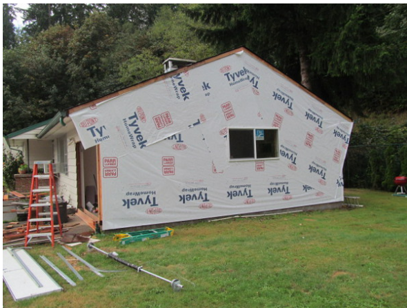
Conference room rehab in progress. USFWS: S. Gronbach
