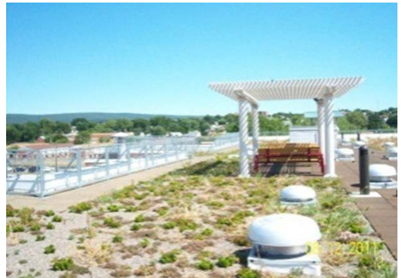
Figure 1: Mountain View's green roof with vegetation and useable terrace space for residents.
