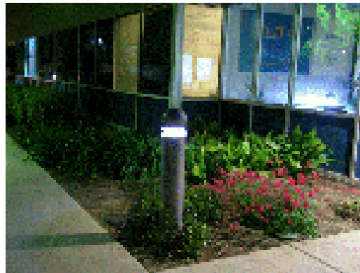
Bi-level LED bollard at the CLTC
