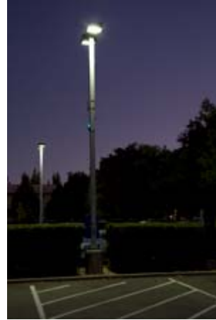
Bi-level induction area luminaire at the California Department of Public Health
