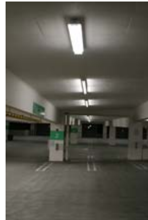
Bi-level fluorescent parking garage luminaire at the University of California, Santa Barbara
