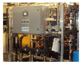
Wastewater recycling system control panel
