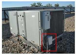
12.5-ton, two-stage RTU at an office building in Beltsville, MD, after installing the Hardware SMDS (outlined in red)
