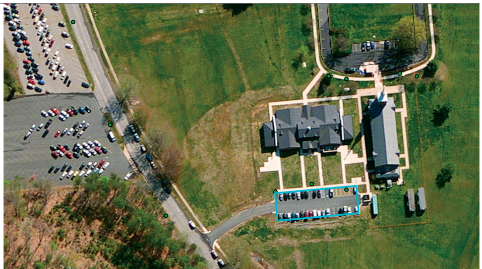
This aerial photo of the Marine Corps Base Quantico (MCBQ) shows the site of the 9,800-ft 2 parking lot (outlined in blue) where mercury vapor fixtures were replaced with LED fixtures, resulting in an energy savings of 85%. Photo courtesy of MCBQ.
