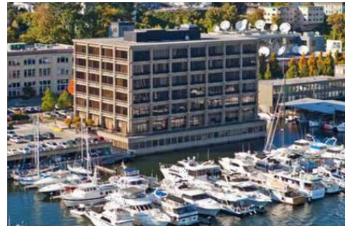
Lake Union Building
