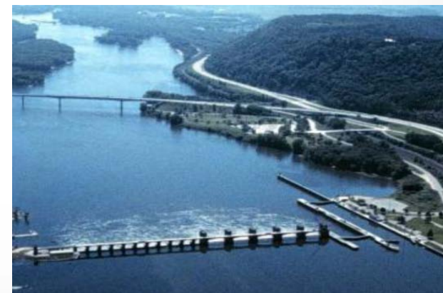
Hydro - low head kinetic Lock & Dam #7, La Crosse
