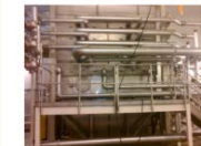
Pipe Insulation - Steam and Condensate Piping (Tulare)
