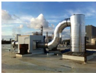
Two Coil Condensing Boiler Flue Gas Economizer - (Melrose)
