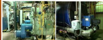
Carlisle - New Burners and Controls
