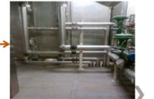
Pipe Insulation - Steam and Condensate Piping (Tulare)
