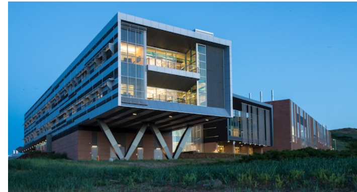
Energy Systems Integration Facility
