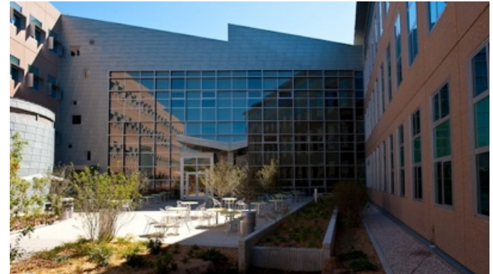
Research Support Facility
