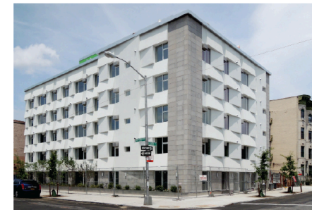
Knickerbocker Commons, the first mid-sized apartment building designed to Passive House standards in the United States
