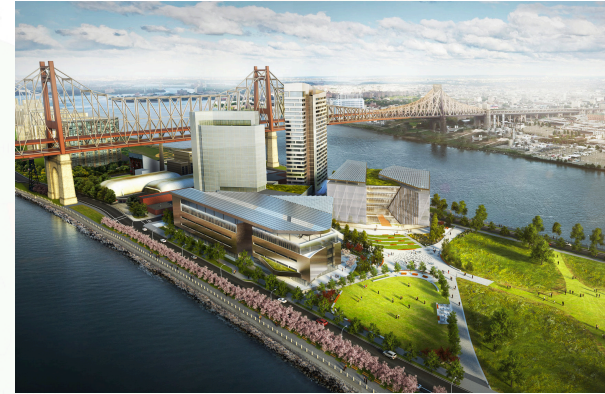
Ground has been broken for a passive-house apartment tower on the Cornell Tech campus on Roosevelt Island. Ruth Fremson/The New York Times
