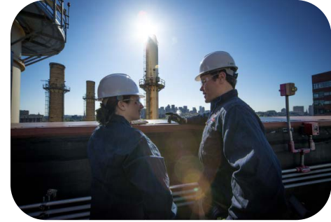
Combined Heat & Power
