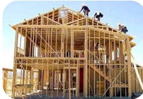
Building Energy Codes
