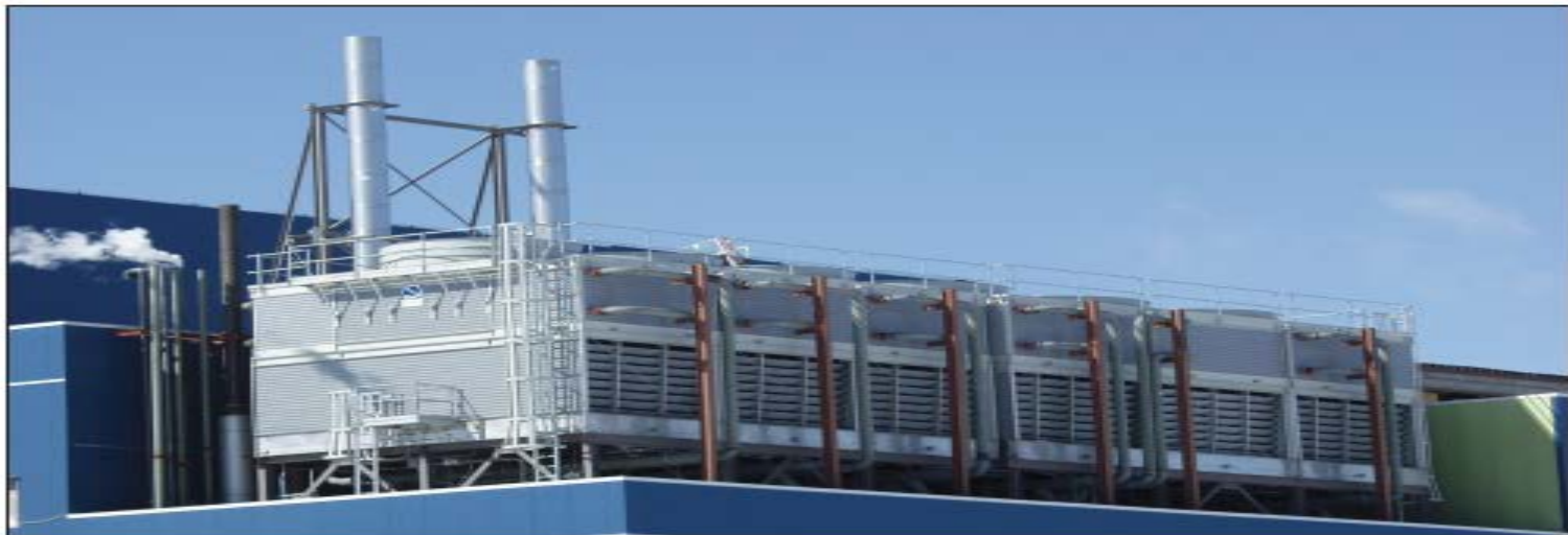
Multi-cell FXV Dual Air Intake Installation
