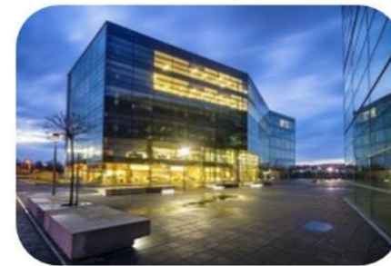
Lighting and Electrical
