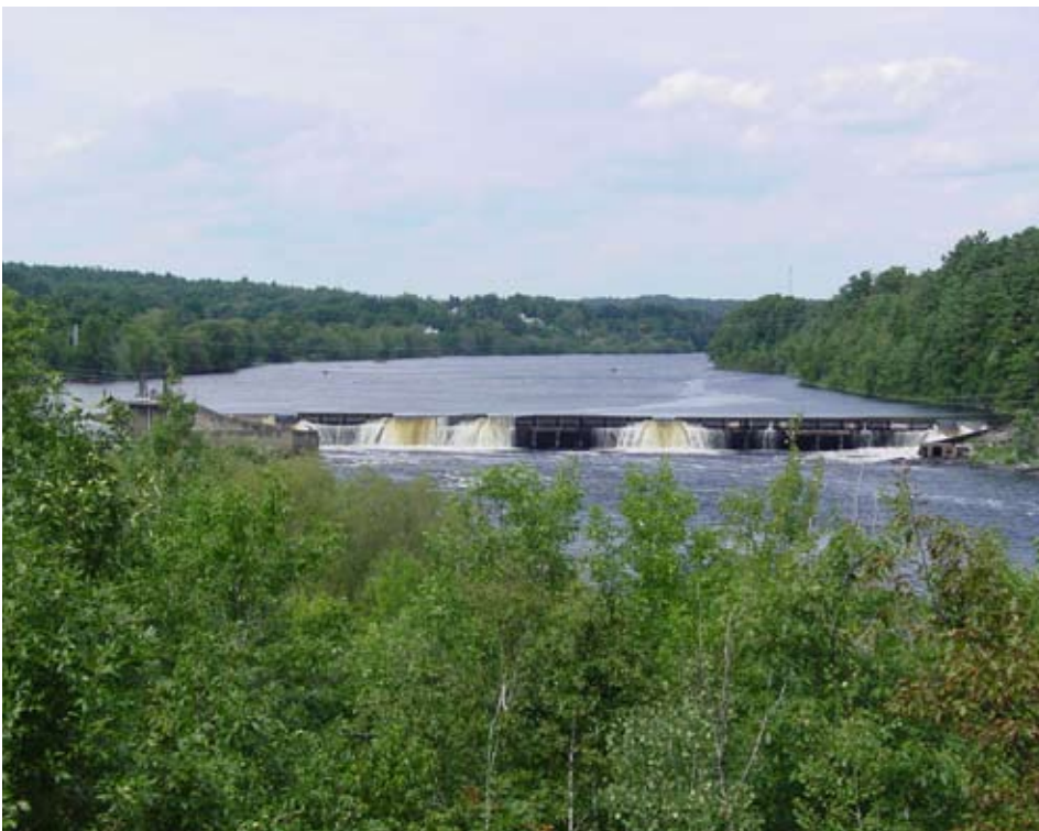
Removal of the Veazie Dam will help to restore fish habitat on the Penobscot River.
