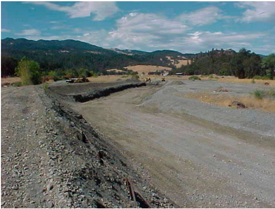
Reconstruction of the Mill Creek channel in 2005.
