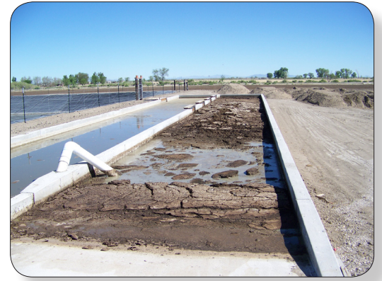
Two large settling ponds catch the waste water from the milking parlor to separate the solids.
