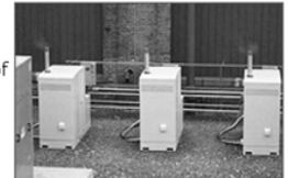
Hydrogen PEM fuel cells are leading candidates for use in fuel cell vehicles. Today's commercially available PEM fuel cells are particularly appropriate for low-power applications requiring intermittent backup.
