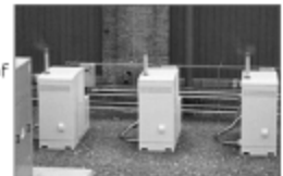
Hydrogen PEM fuel cells are leading candidates for use in fuel cell vehicles. Today's commercially available PEM fuel cells are particularly appropriate for low-power applications requiring intermittent backup.
