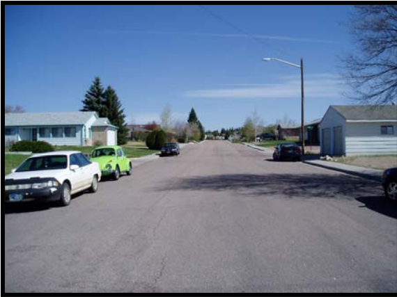
Recent Subdivision Street – No Street Trees
