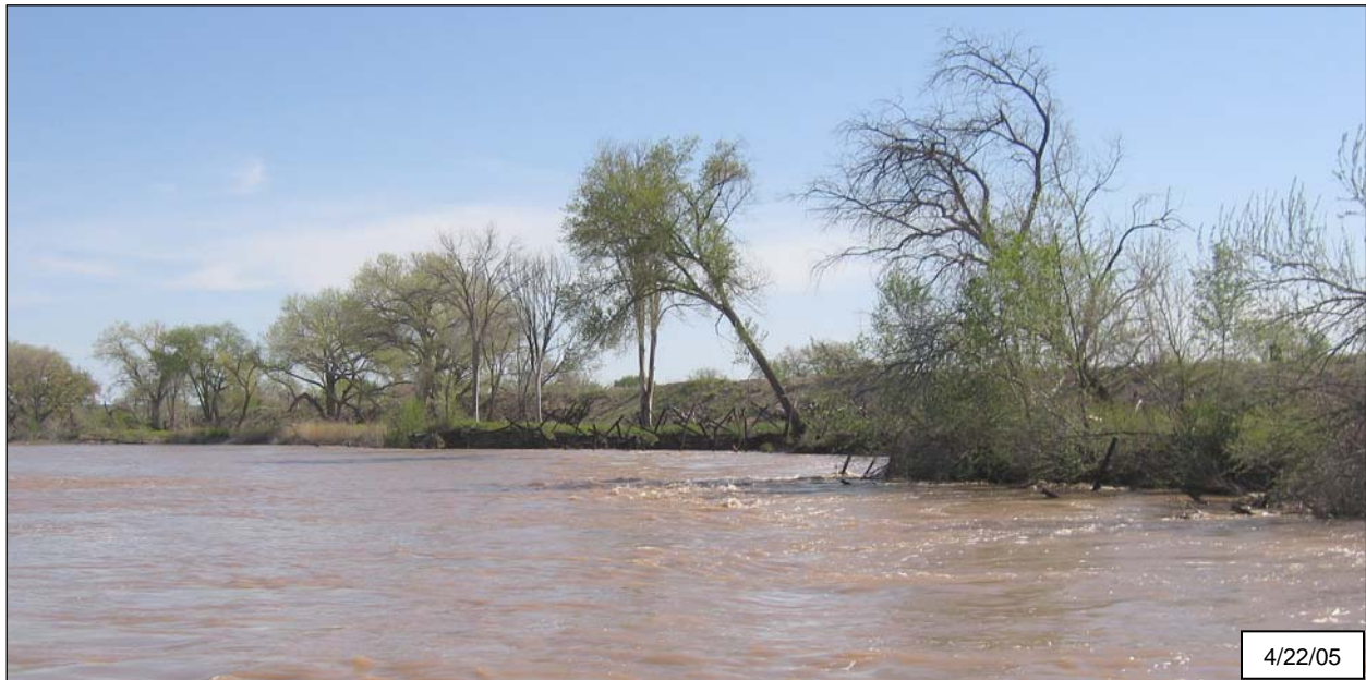
Figure 4: Bank erosion/bend migration at the Bernalillo Priority Site on April 22, 2005.
