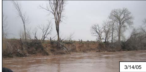
Figure 3: Bank erosion just downstream from the rip-rap armoured bankline at the Bernalillo Priority Site.
