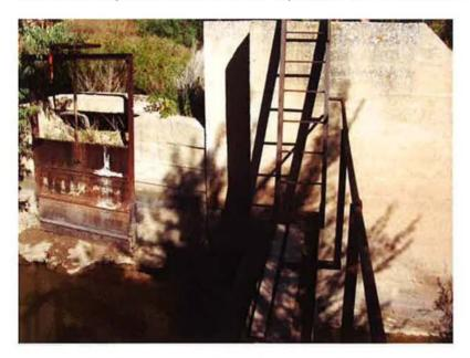
Photo 1: This is the existing diversion structure at Cottonwood Creek (left bank) that corresponds with the northwest beginning of the State Road Canal. This diversion structure would be modified to divert waters into the proposed settling basin. The proposed settling basin would supply the proposed State Road piping system.
