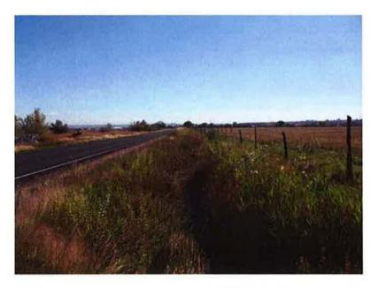
Photo 17: This photo captures the Martin Lateral along 2000 South, east of 4000 West. The proposed piping alignment is located in this existing/established irrigation ditchline. Post piping installation, a roadside swale would be cut into this area to handle roadway stormwater and irrigation run-off waters.
