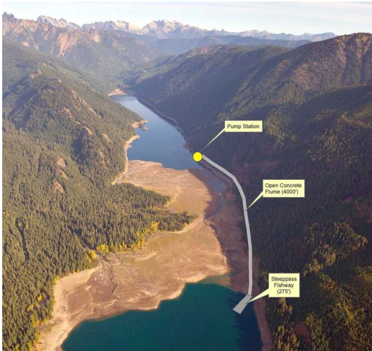
Figure 9-30. OPTION 5 - The Narrows: Lower to Upper Reservoir Passage - Electric Pump conceptual drawing.
