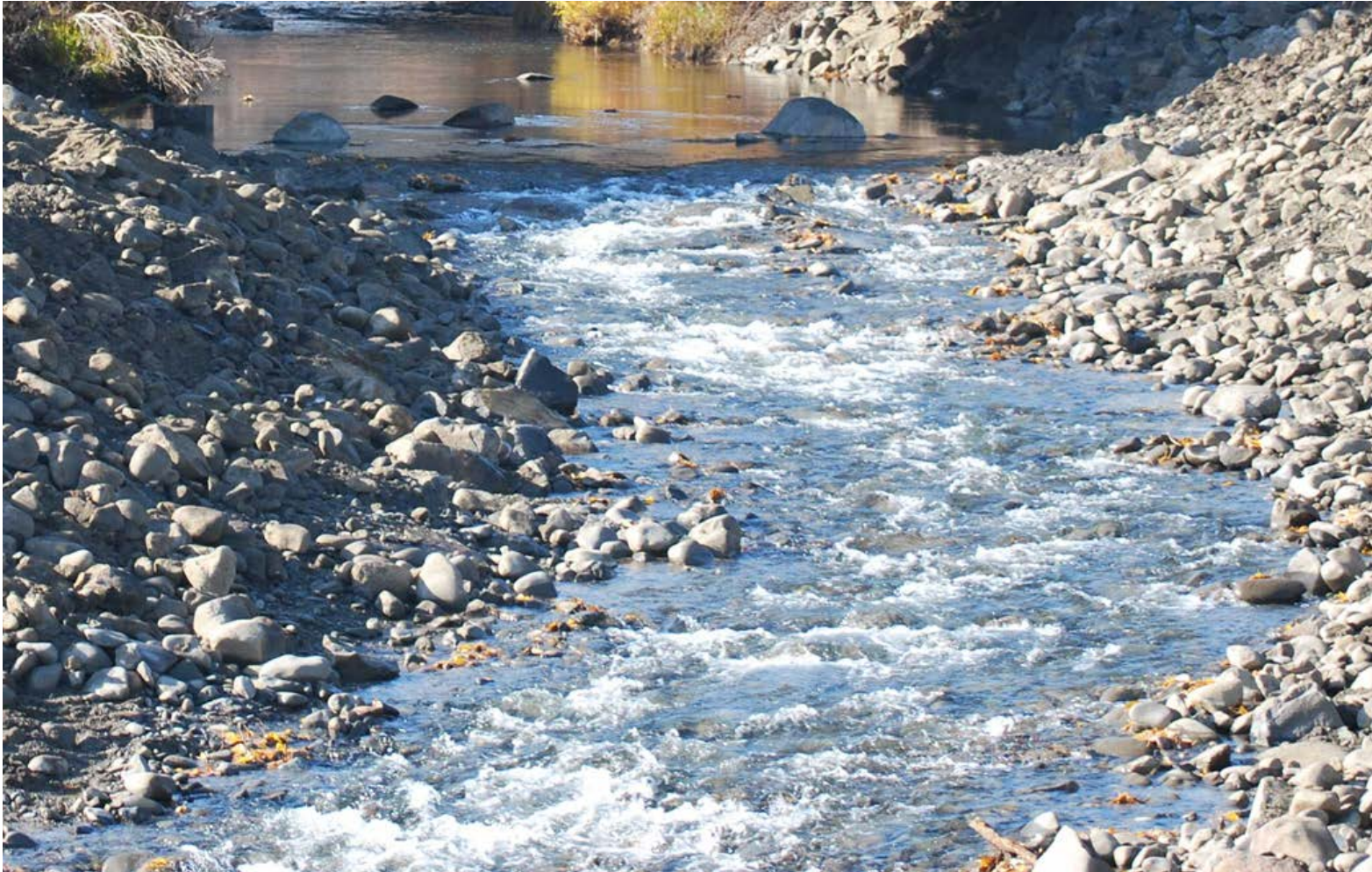
Figure 9-25. OPTION 2 – Box Canyon Roughened Channel would be designed similar to the Bruton channel on lower Taneum Creek above .
