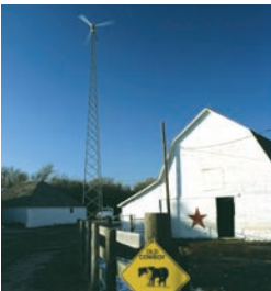
Location — A farm in western Kansas Capacity — 10 kilowatts Turbine manufacturer — Bergey Windpower Company Photo credit — Warren Gretz, NREL/PIX09618
