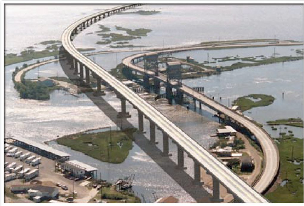
1 2 Figure 25.5: Adaptation Possibilities for Coastal Infrastructure
