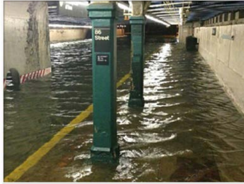
Hurricane Sandy Causes Flooding in New York City Subway Stations
