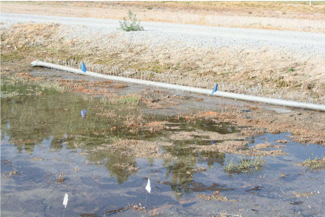
Perforated irrigation pipe watering the pond.
