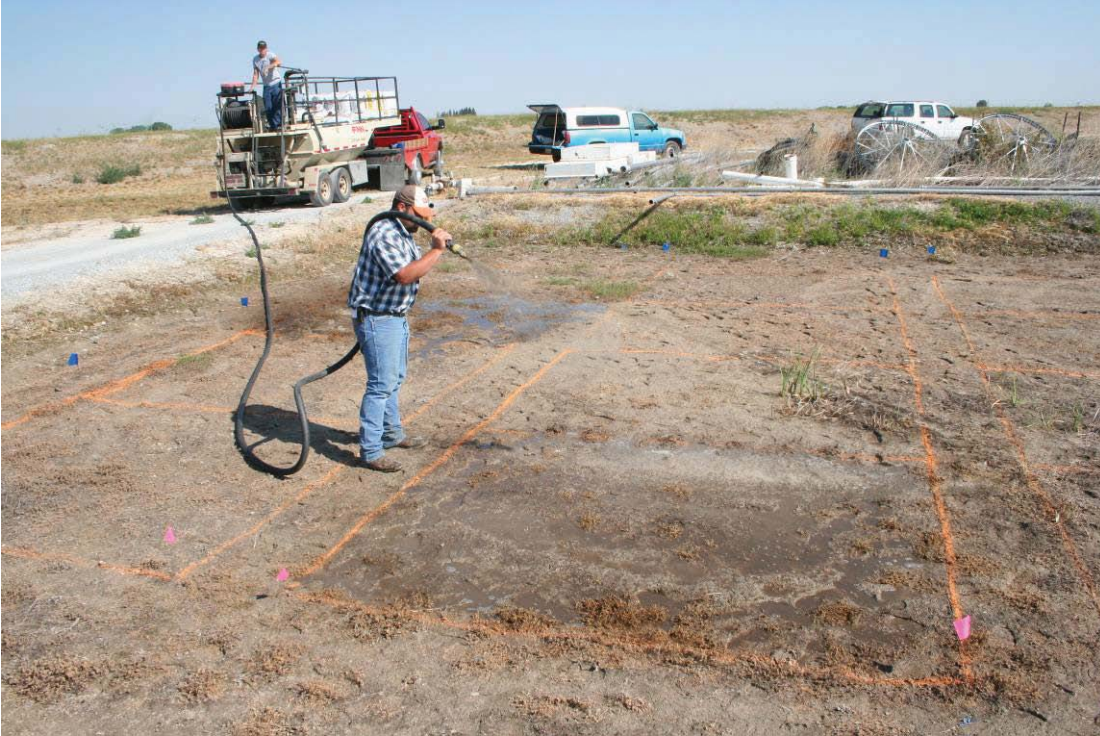
Hydroseed application of Fertil Fibers treatment.
