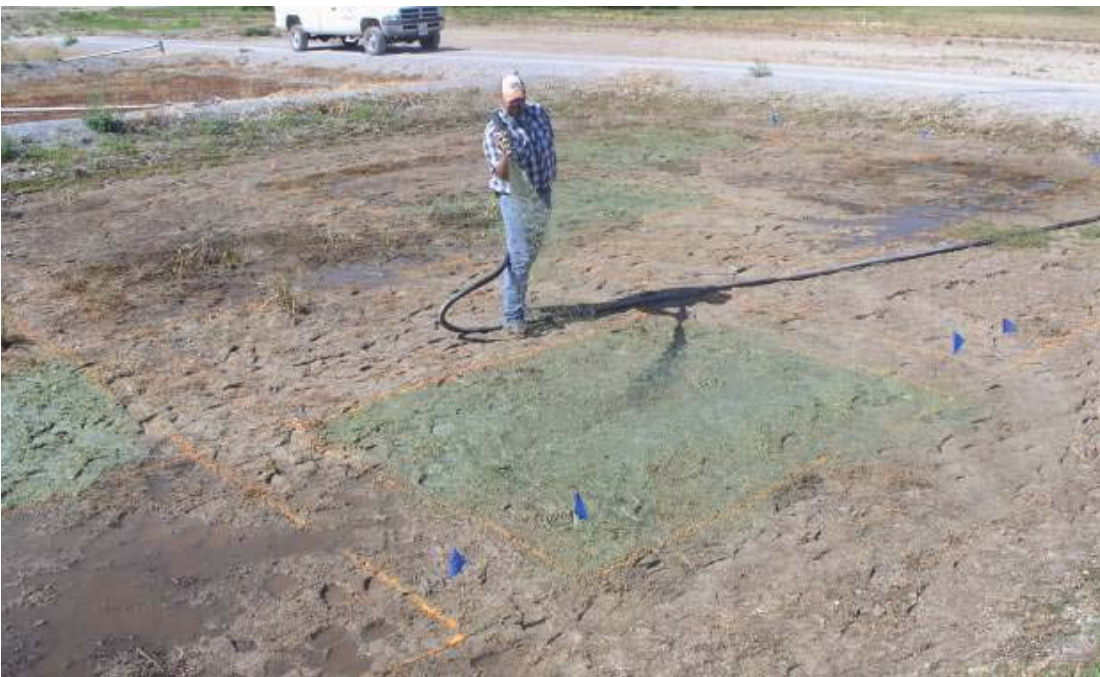
Hydroseed application of Fertil Fibers and straw mulch treatment.
