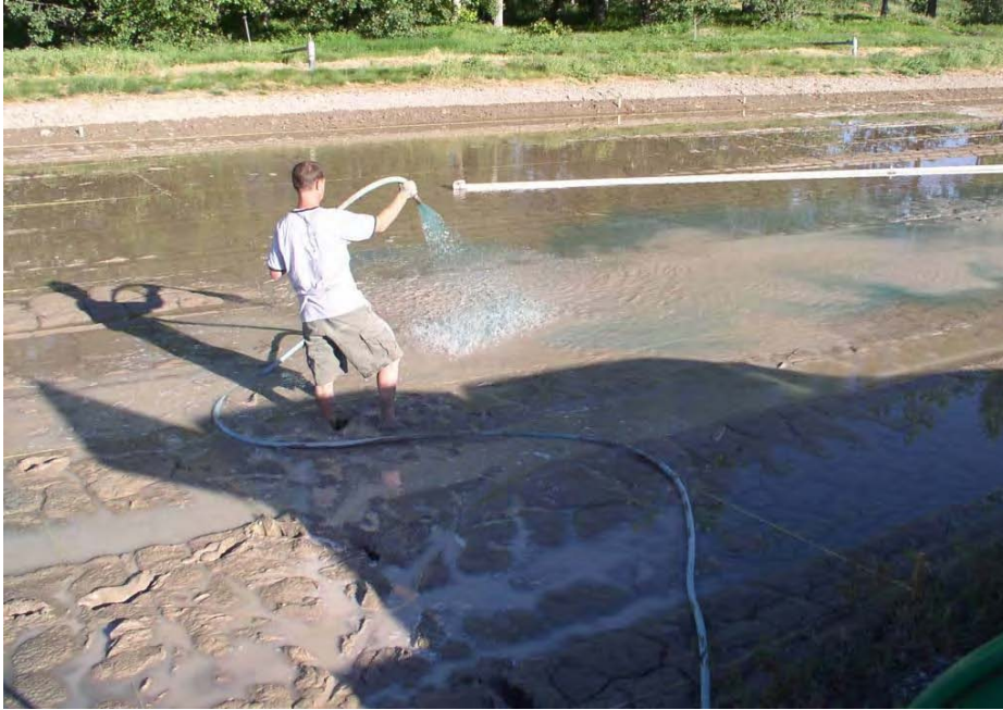
Figure 2. Hydroseeding into slurry prepared pond. The hydroseed mixture sank into the water and settled on the muddy surface.
