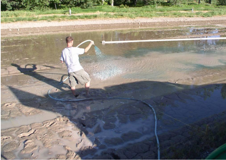
Figure 2. Hydroseeding into slurry prepared pond. The hydroseed mixture sank into the water and settled on the muddy surface.
