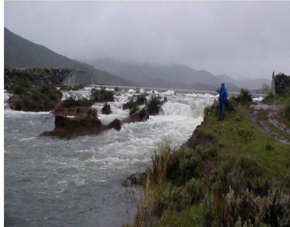
Little Wood Reservoir spillway in central Idaho May 18, 2005 after two inches of rain fell in one day on top of a ripe snowpack.
