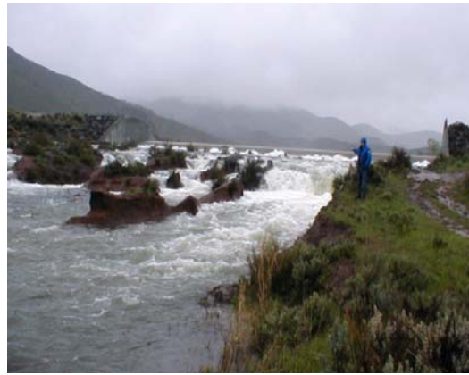
Little Wood Reservoir spillway in central Idaho May 18, 2005 after two inches of rain fell in one day on top of a ripe snow pack
