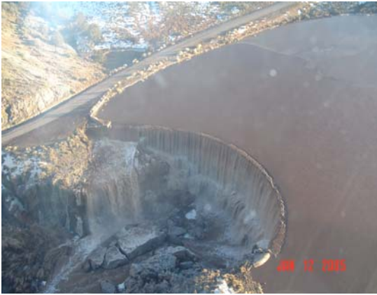
Lower Enterprise Dam southern Utah January 12, 2005 after a heavy precipitation event
