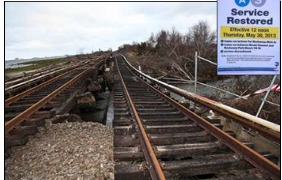
Repaired MTA A Train track at the Rockaways
