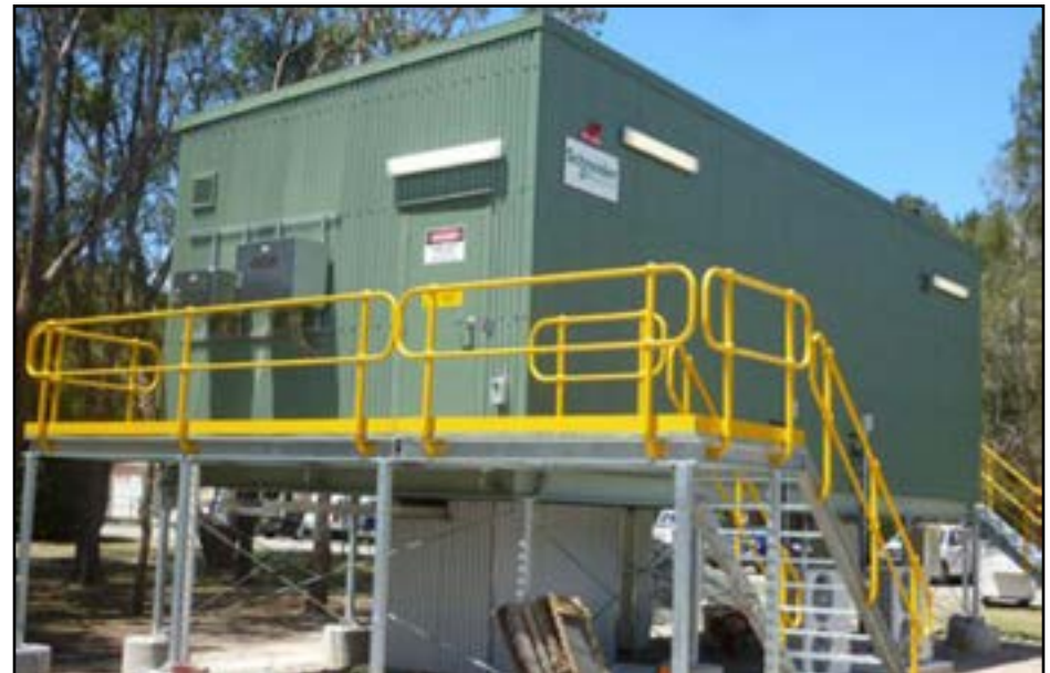
Elevated Facility Structure
