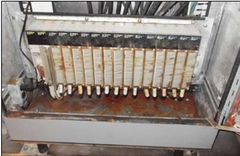
Storm Debris in South Ferry Station
