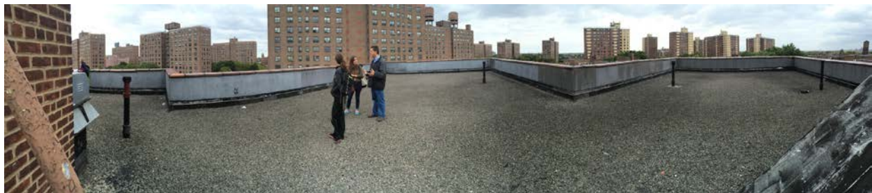
Figure 20. Roof of the NYCHA Senior Center/Cooling Center looking south
