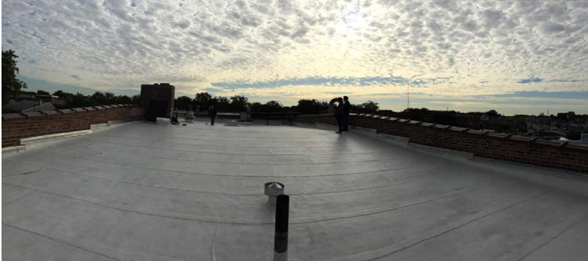
Figure 14. Roof of the fire station looking east from the west side
