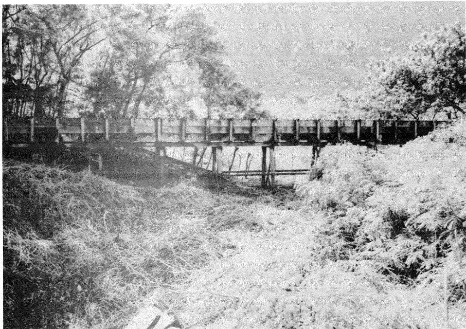
PHOTO NO. 7 - Waimanalo Irrigation System flume and trestle at a typical foothill stream crossing in the irrigated area.
