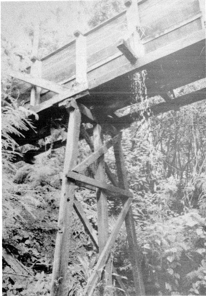
PHOTO NO. 6 - Waimanalo Irrigation System flume and trestle in the irrigated area.
