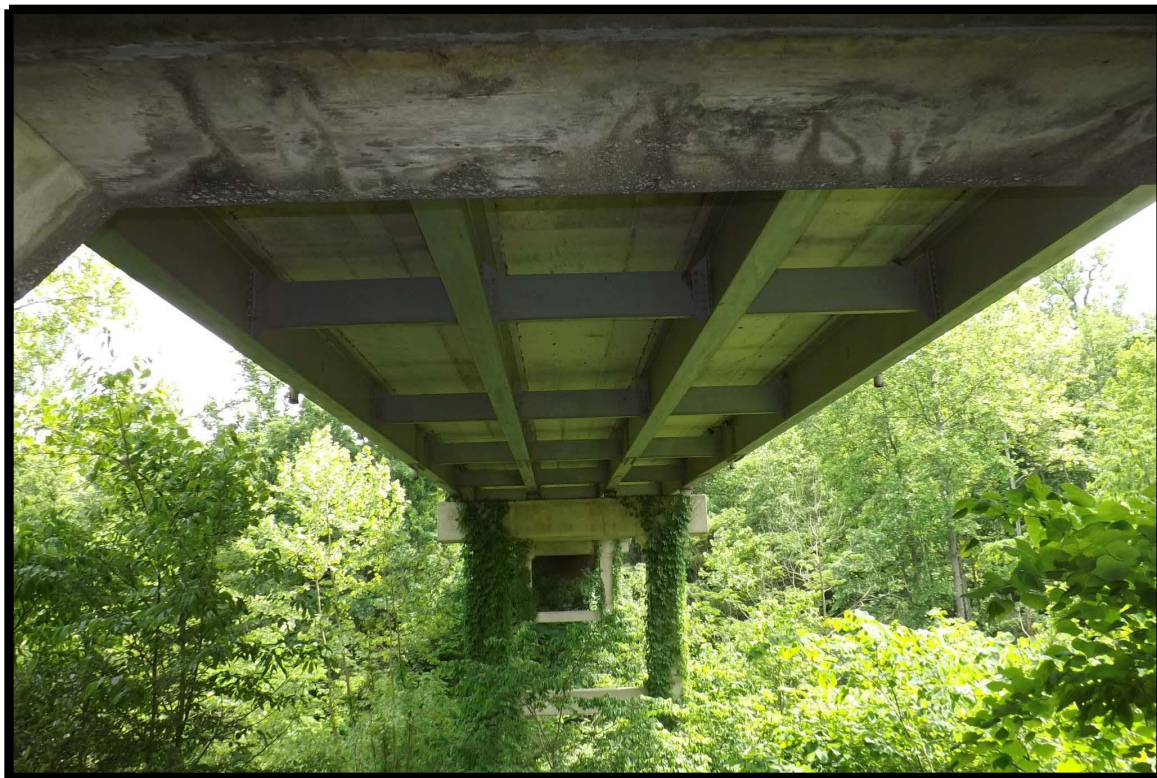
Typical view of underside of bridge
