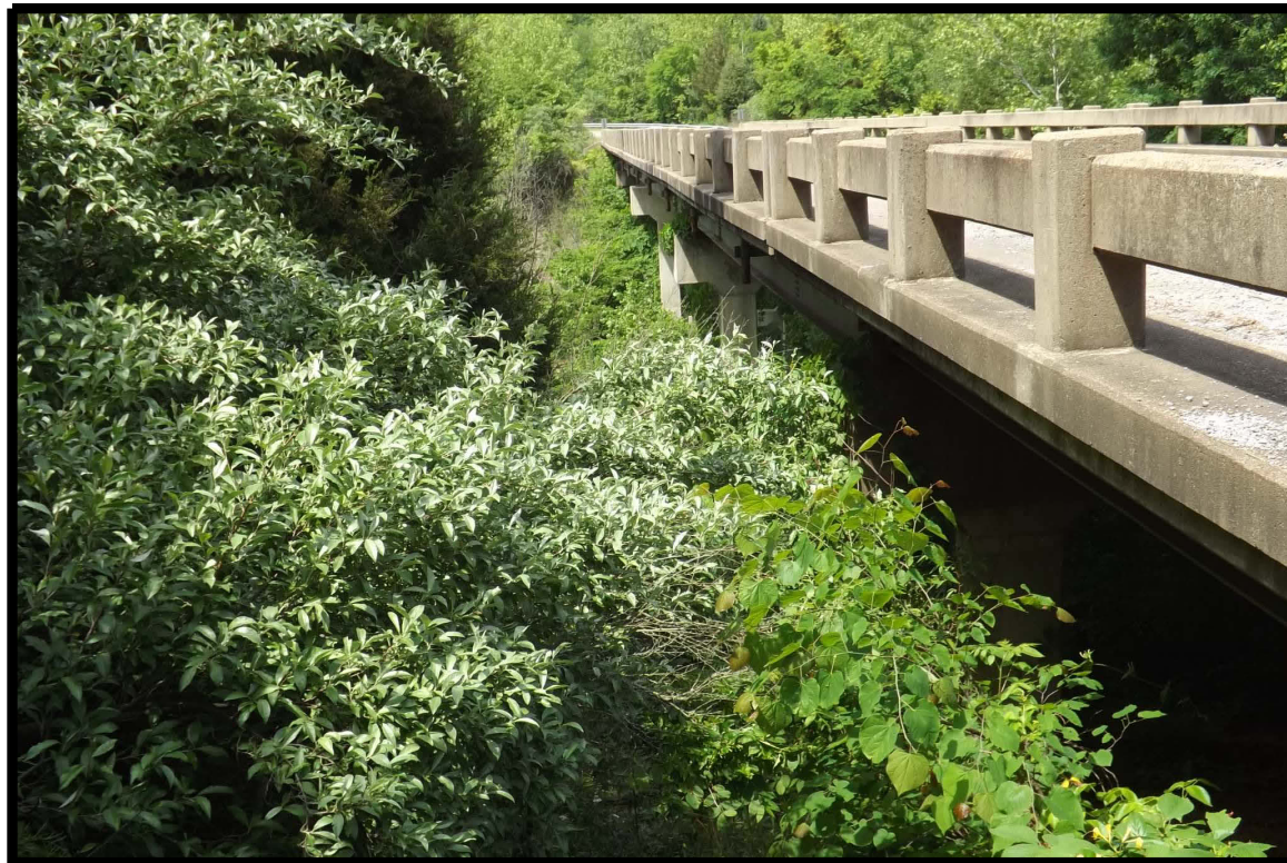
Side view looking downstream
