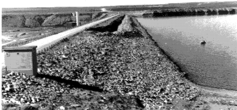
Fontenelle Dam and Reservoir.
