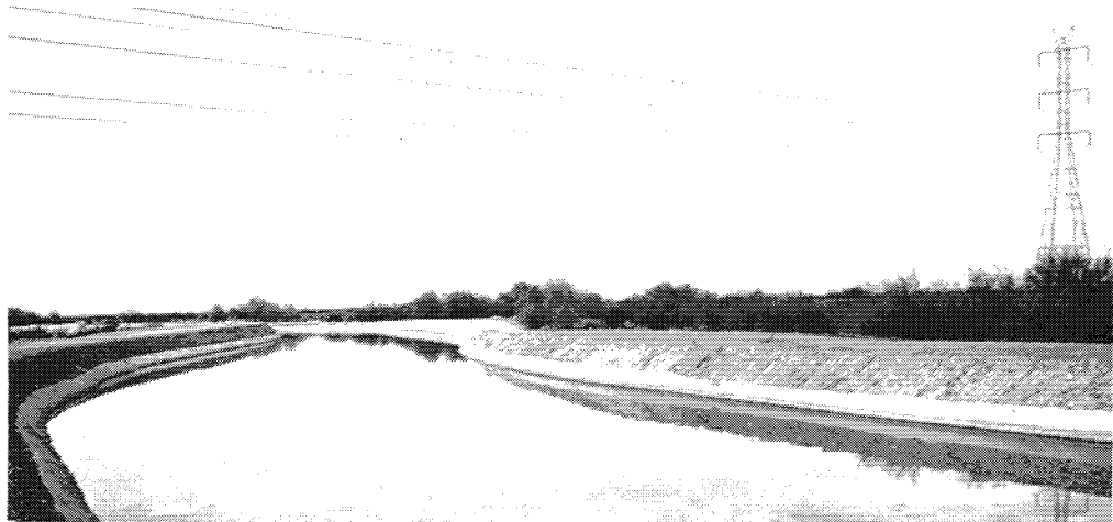
Canal lining reduces seepage losses.
