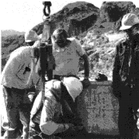
Rigging of bosun chair used for dam inspection.
