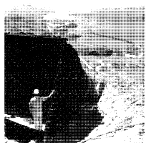
Pipeline at Havasu Pumping Plant.
