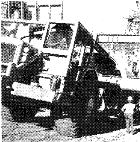
Pipeline emplacement equipment.
