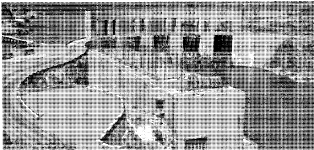
Parker Dam and Powerplant, Ariz.
