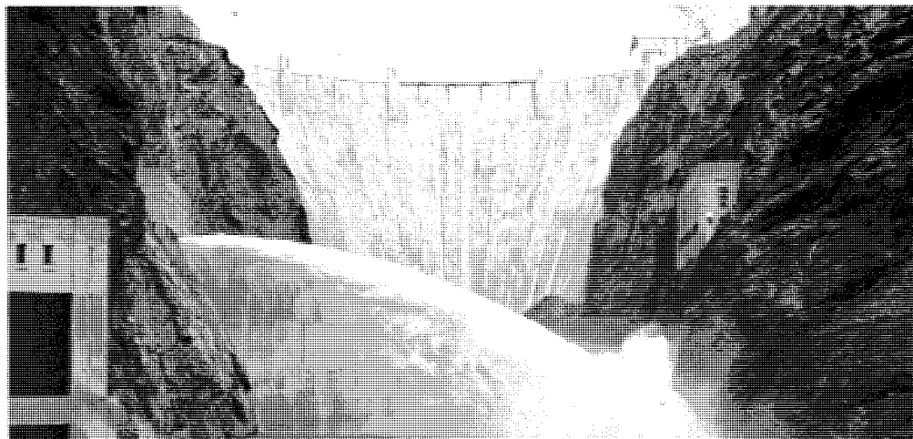
Hoover Dam, penstock flushing, Nev.-Ariz.
