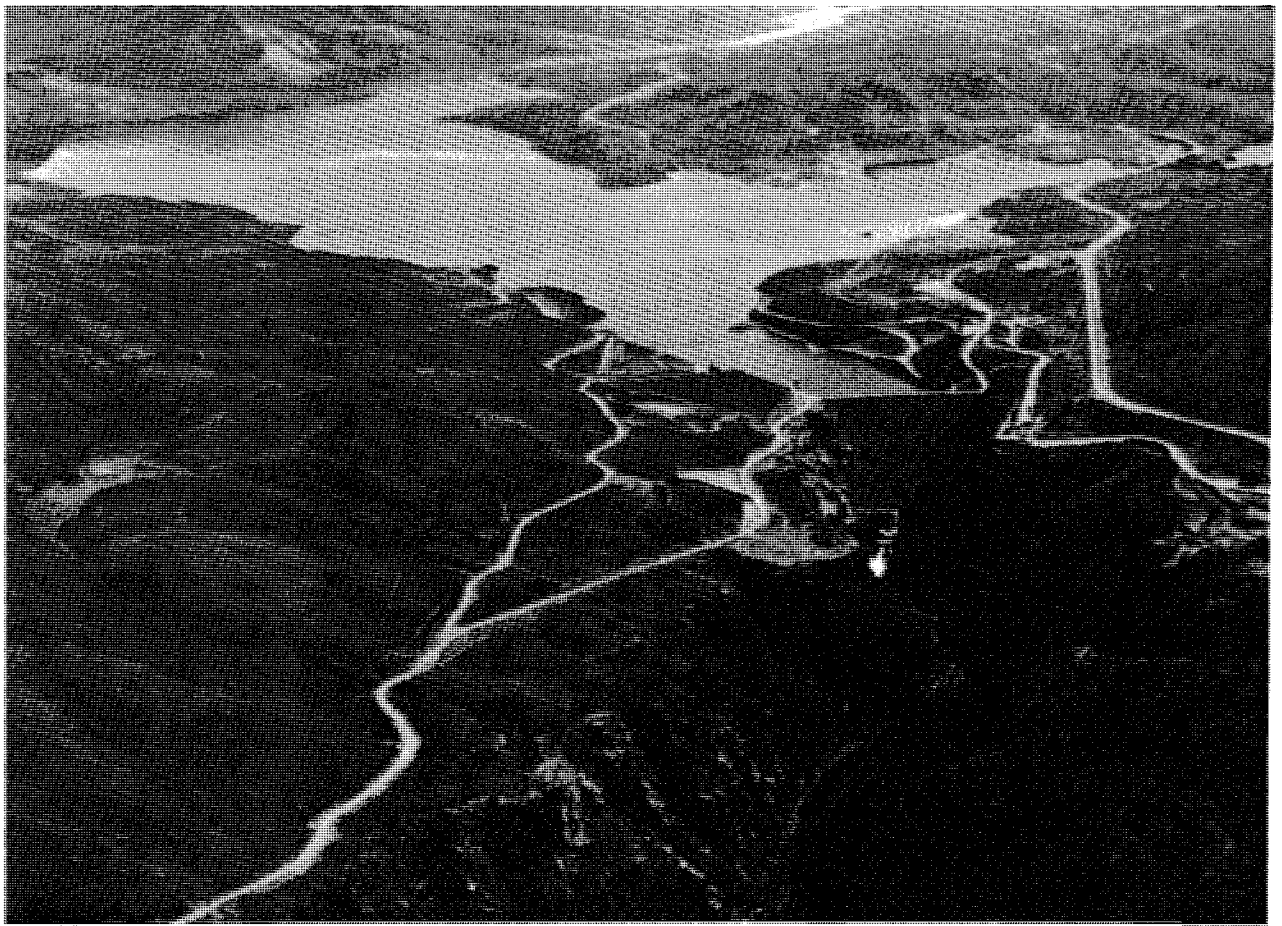
Blue Mesa Dam, Curecanti Unit, Colorado River Storage Project, Colorado.
