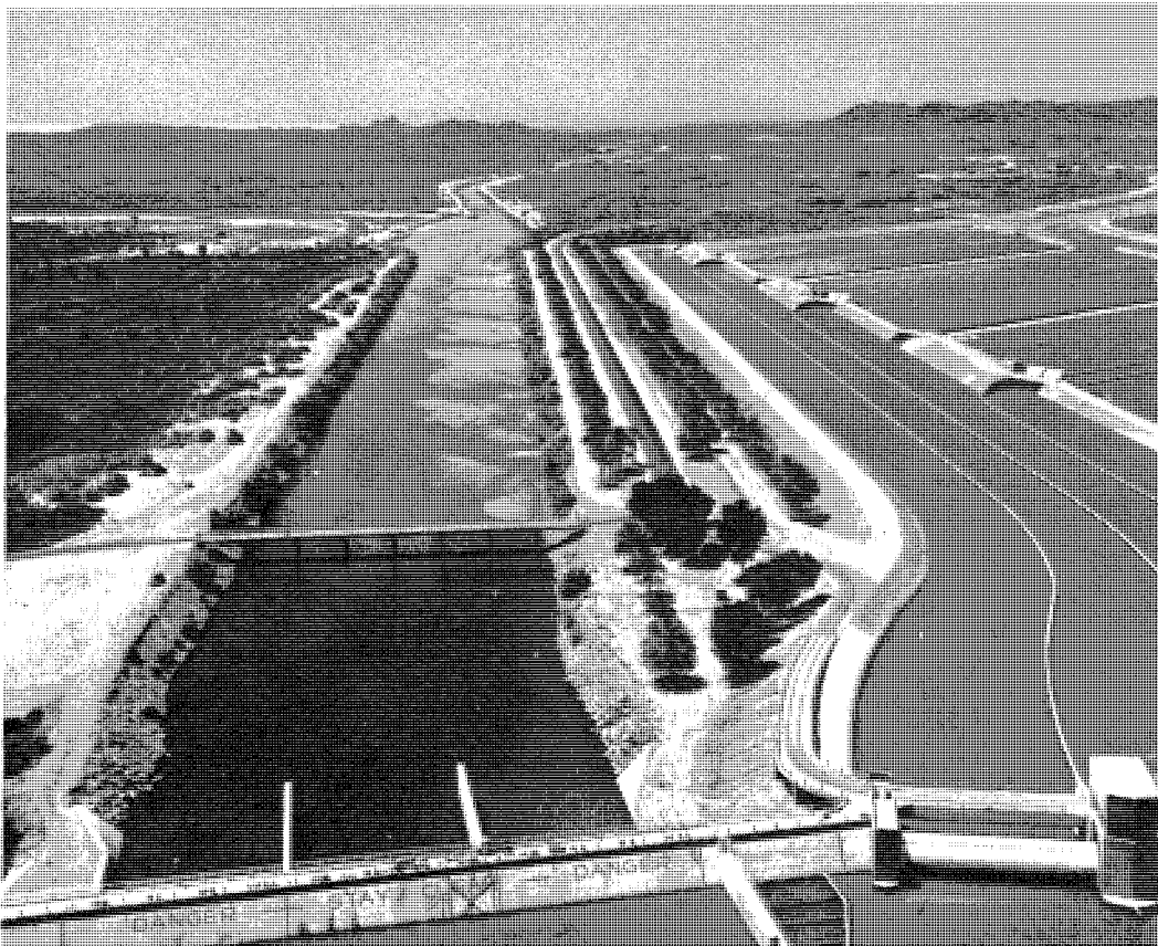
Looking south from Imperial Dam, left to right, the California Sluiceway, All-American Canal, and the Desilting Basins, California.
