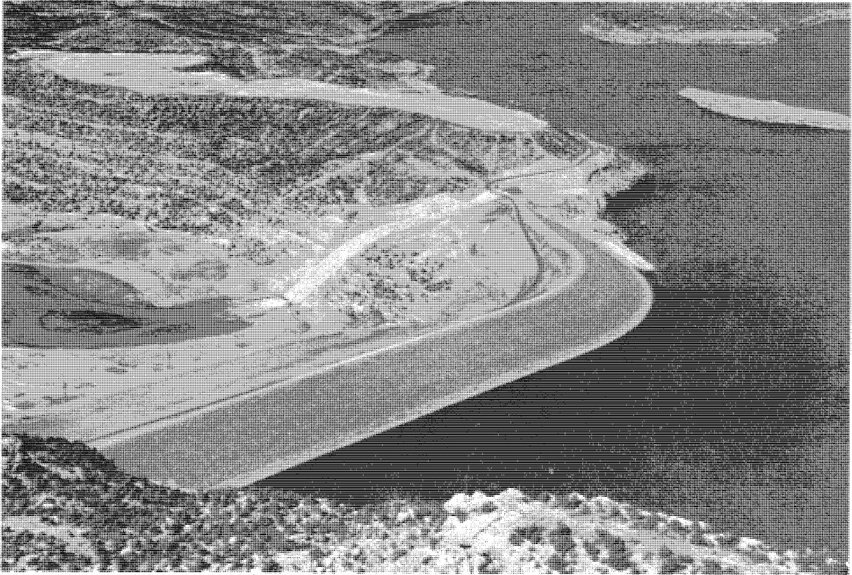
Navajo Dam and Reservoir, Navajo Unit, Colorado River Storage Project, New Mexico-Colorado.
