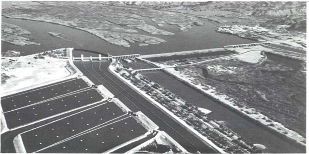
Imperial Dam and desilting works, Arizona-California
