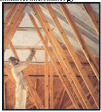
Many interior coating products have names that sound like a radiation control coating, but unless the label shows the emittance is between 0 and 0.25, they won't perform as intended.
