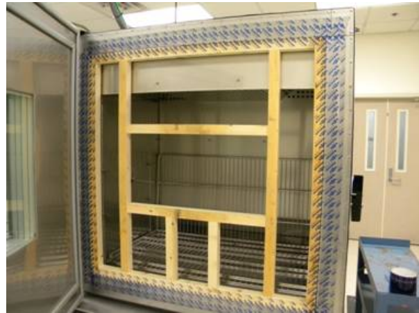
Figure 13. Framing for climate chamber opening
