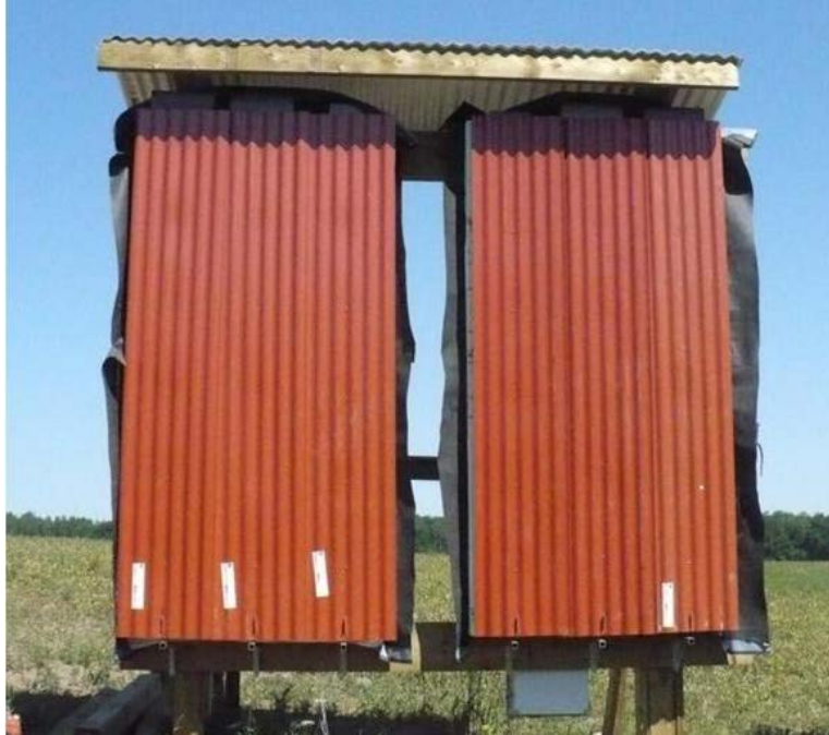
Figure 22. Lightweight cladding panel installed over the test wall assemblies
