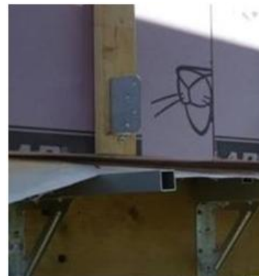
Figure 23. Deflection measurement location
