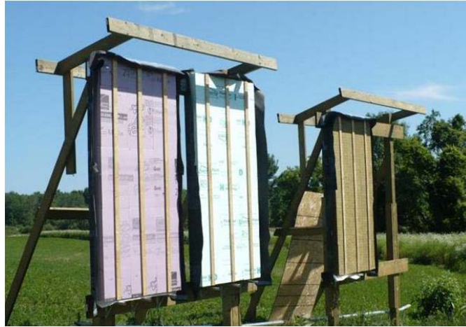
Figure 20. Test wall assemblies under construction
