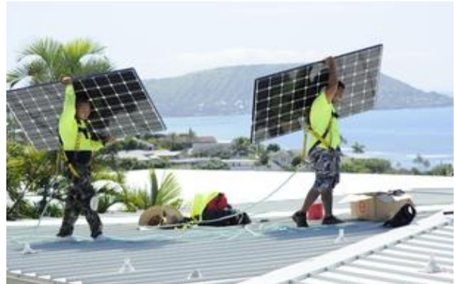
Hawaiian Electric employees installing rooftop solar.
