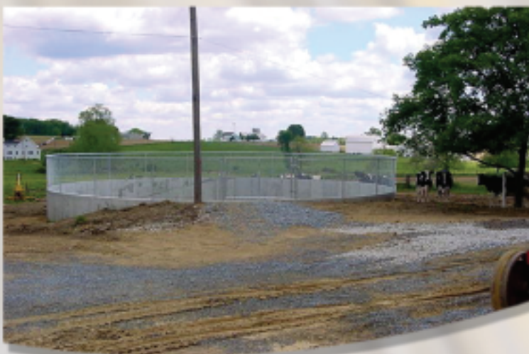
Manure storage facilities prevent runoff and the contamination of surface and groundwater.
