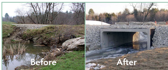
Replacement of culvert that blocked smelt from spawning habitat. USDA
