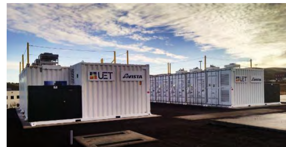
UET vanadium flow battery in Avista, Washington
